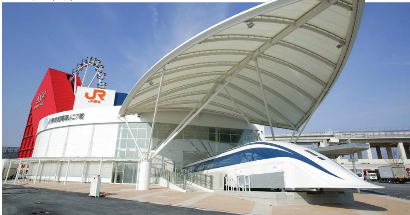
JR Central Pavilion
